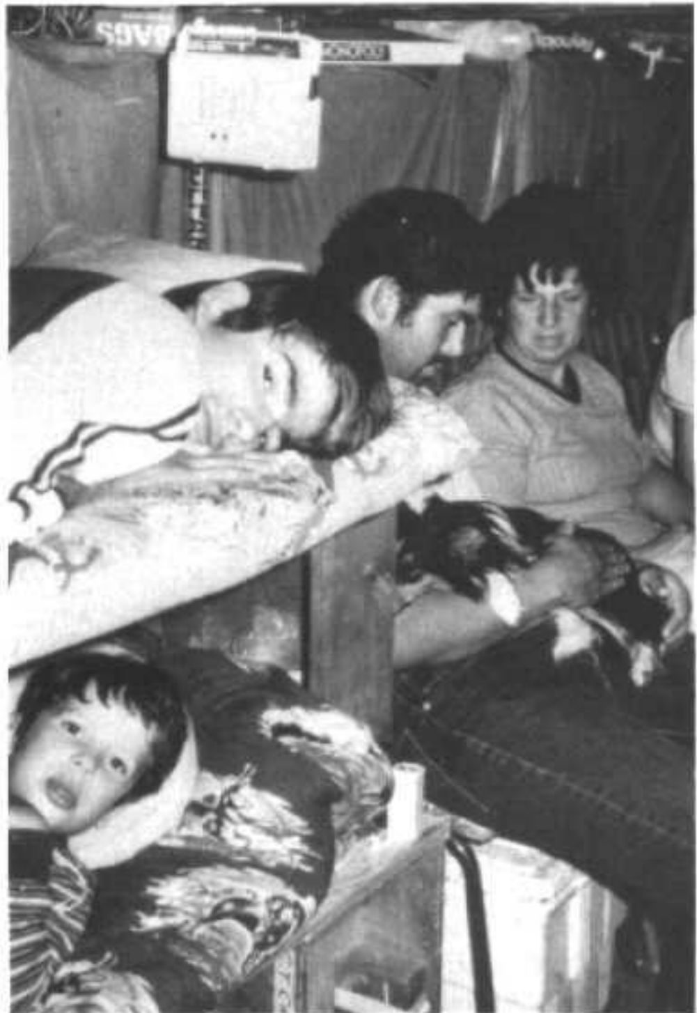
Fig. 14.2. Benches with overhead bunks in a skillfully designed Small-Pole Shelter of Russian design. Three rural families in a wooded area of Tennessee built this expedient blast shelter in 48 hours, including the time spent felling trees and making furnishings.
