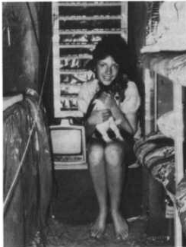
(Photograph) Fig. 6.2. Behind the girl is the homemade air pump that made it possible for a family of six to live in a crowded trench shelter for more than three days. Outside the temperature rose to 930 F.
